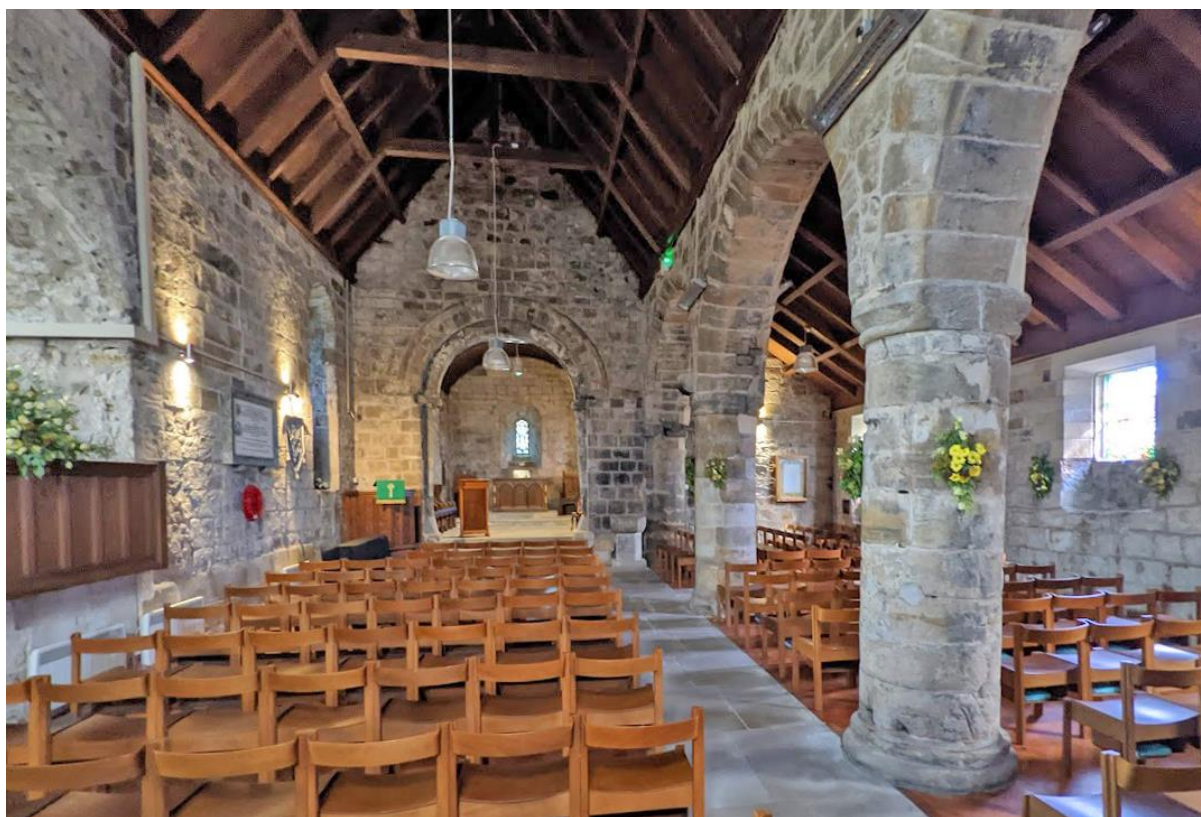
Interior looking east
