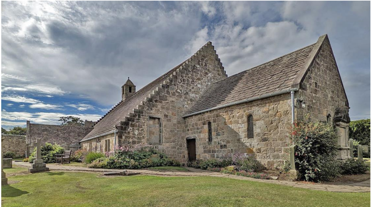
The church from the south east
