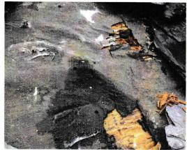
We have carried out an investigation of the hall roof and have drawn up a schedule of necessary major repairs to be carried out urgently with our chosen roofing contractor. During this investigation the sarking was found to be rotten on the north elevation round the perimeter of the roof and the east hall roof was found to be in poor condition.
